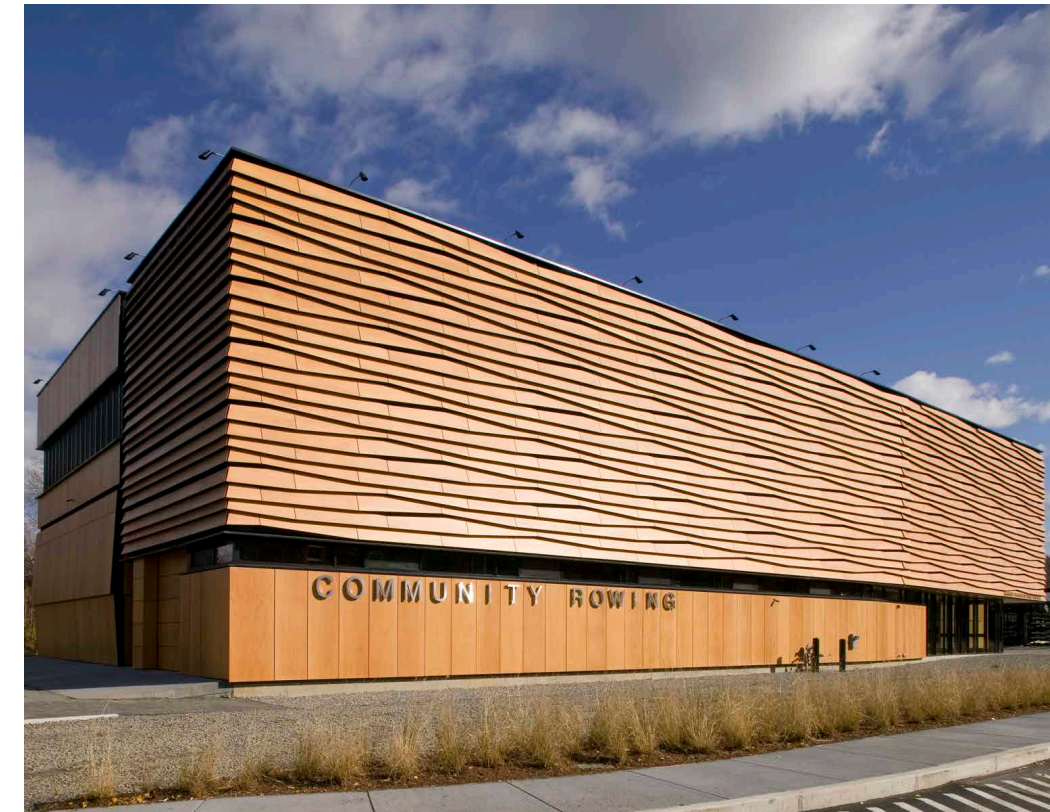
A custom designed Prodema panel facade for the Harry Parker Boathouse in Brighton, MA. Designed by Anmahian Winton Architects, and winner of the 2014 AIA Honor Award for Architecture
