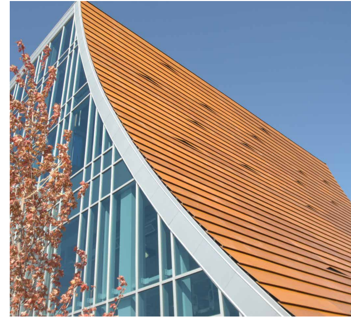
A custom designed Prodeema panel facade for the UNO School in Chicago. Designed by UrbanWorks, Ltd. Winner of the 2013 ALA Award for Gold Medal Design
