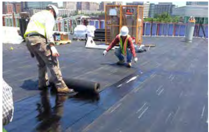
Installing Hydroflex protection sheet (RB II or 30) into second layer of MM6125 membrane
