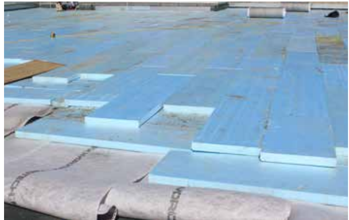
DuPont STYROFOAM® is installed in layers to depth needed to achieve R-rating
