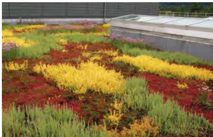
Tri-City Wastewater - Oregon City, OR
