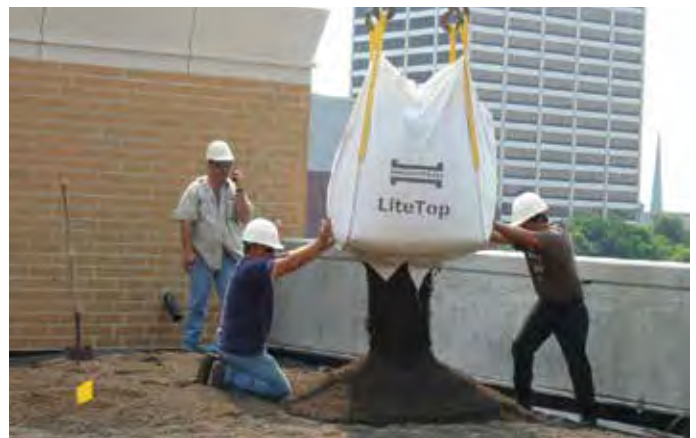
LiteTop® installed to desired depth
