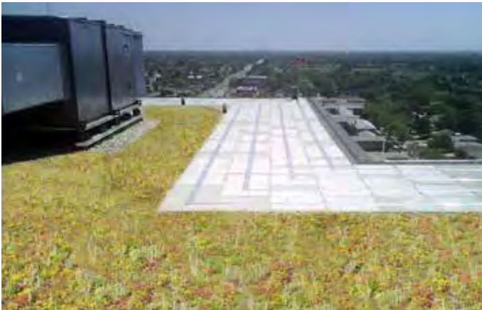
Example of extent of ballast pavers on roof
