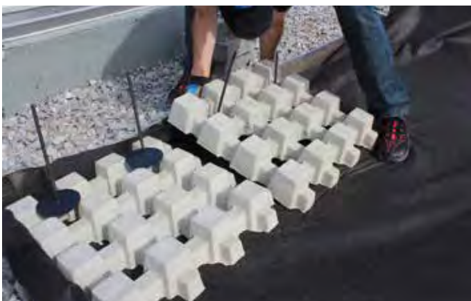
Checker Block® installation on rooftop
