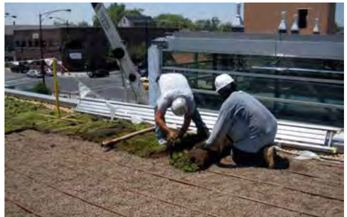
Plant materials being installed over prepared LiteTop®
