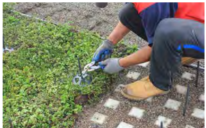
Vegetation installation is completed with trimming of Disk Anchors
