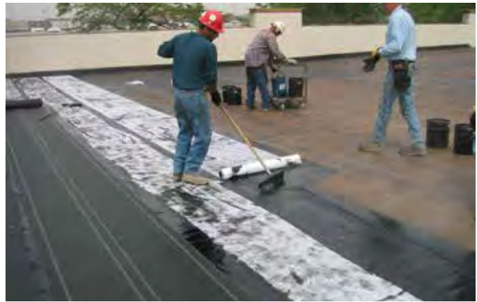
Installing MM6125-FR waterproofing membrane with reinforcing fabric - total thickness of 215 mils
