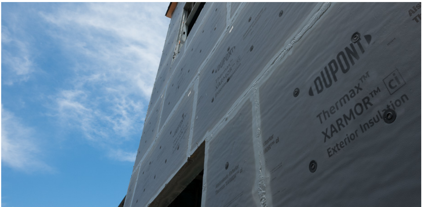
Photo: DuPont™ Thermax™ Wall System using Thermax™ XARMOR™ (ci) Exterior Insulation with DuPont™ LiquidArmor™ Flashing and Sealant applied to board joints.
