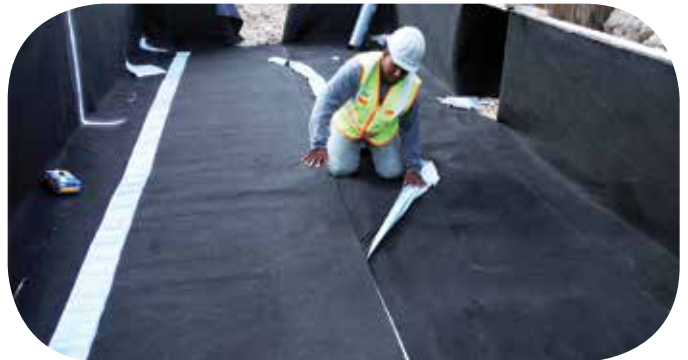
The self-adhering side laps make installation of the Underseal® Underslab Membrane quick and efficient.
