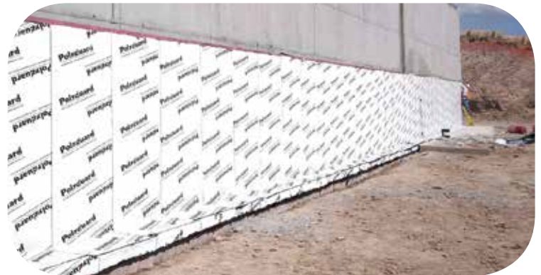
650 Membrane provides continuous waterproofing for concrete foundation walls.
