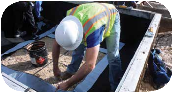
Underslab Membrane being installed to waterproof an elevator pit.
