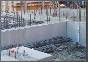
WallGUARD<sup>®</sup> panels are installed using specially designed galvanized steel mounting clips, which are
