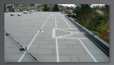
By simply reversing conventional design and placing the insulation above the membrane rather than below, the cause of many life shortening roofing problems can be eliminated. This unconventional arrangement of roofing material—roof deck, roof membrane, LightGUARD® or HeavyGUARD® ballasted roof insulation panels—is commonly referred to as the upside-down system, or Protected Membrane Roofing (PMR) system.
